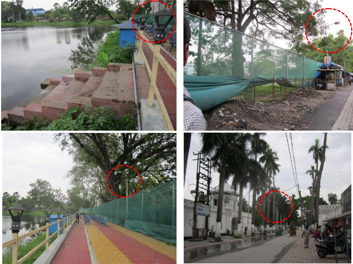
Figure 4: Existing Illumination and electric cables around Bairagi Dighi. A: low height lights along the tank, B, C & D: street lamps (clockwise from top left). Note the overhead cables in image C.
