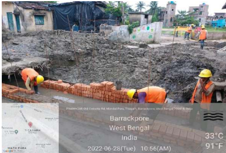
BARRACKPORE STP SITE
