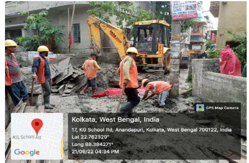
BARRACKPORE STP SITE
