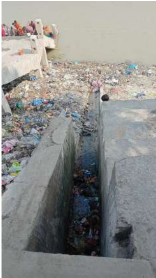
Outfall falling into Ganga
