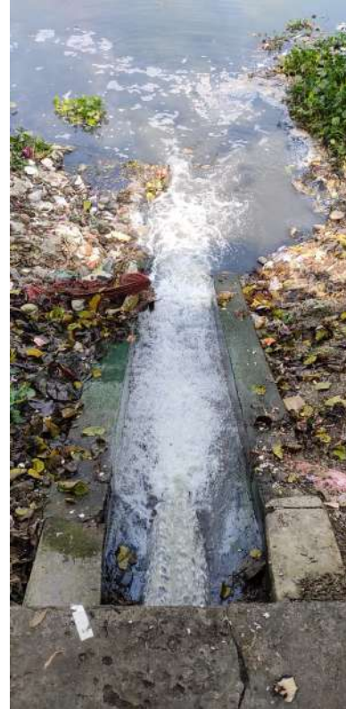
Outfall falling into Jalangi River
