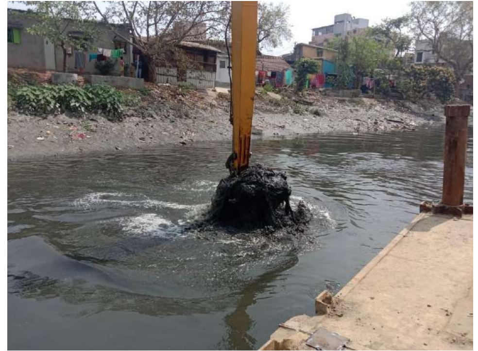
Picture TNP2: Dredging Work at Tolly's Nullah near House of Hon'ble CM
