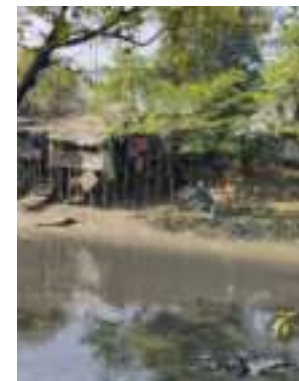
Encroachment on the bank
