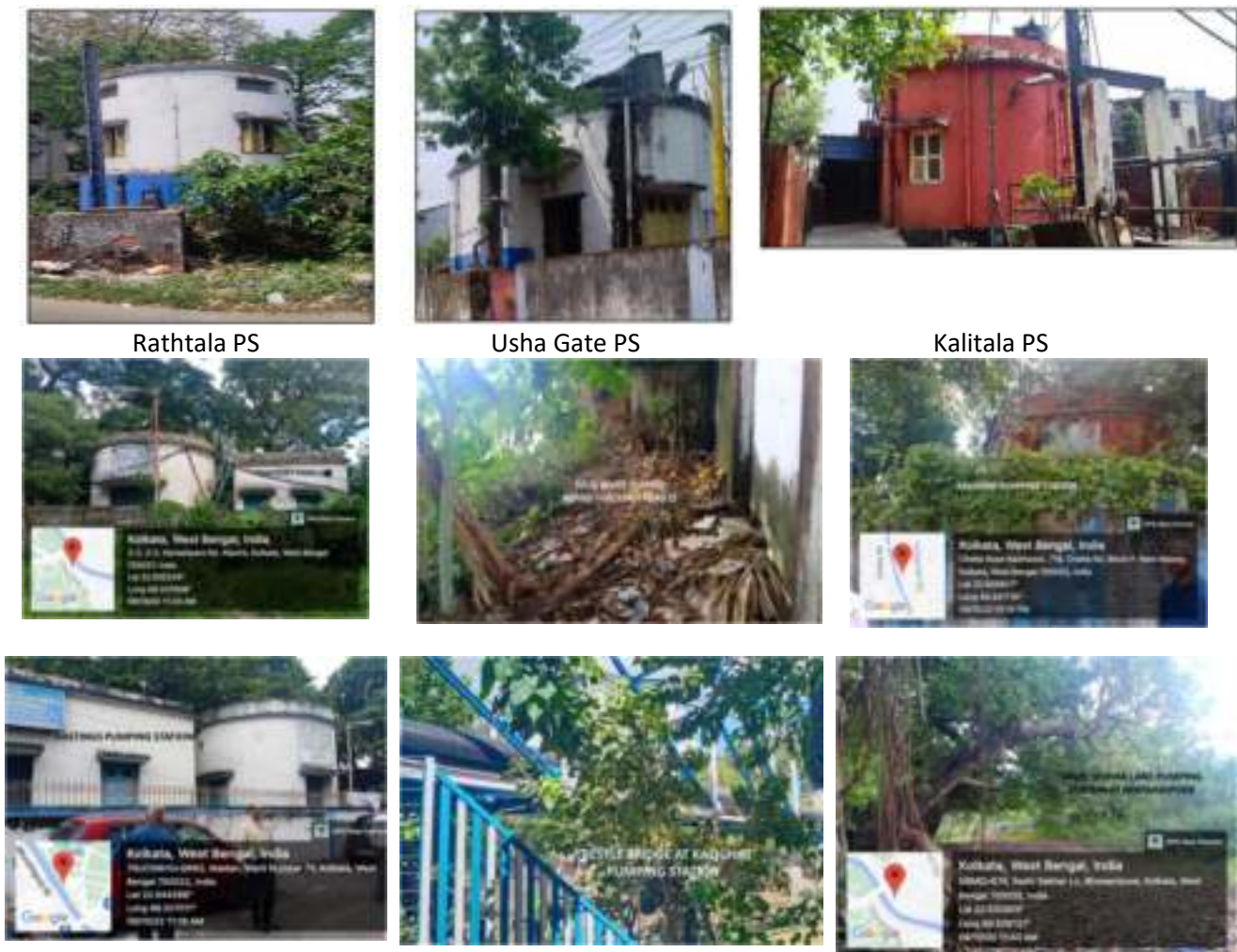
Figure 2-10: Existing lifting / pumping stations of Tolly nullah
