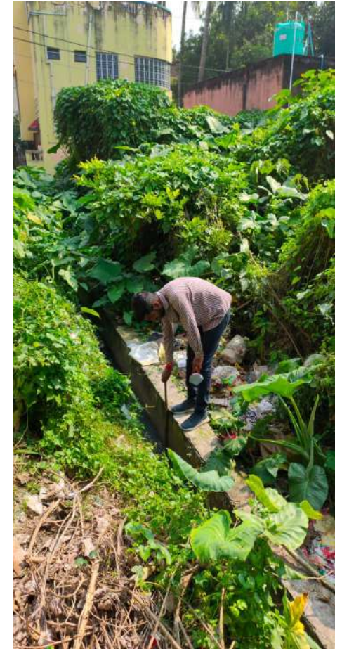
Identification of Outfalls & Flow Measurement Survey
