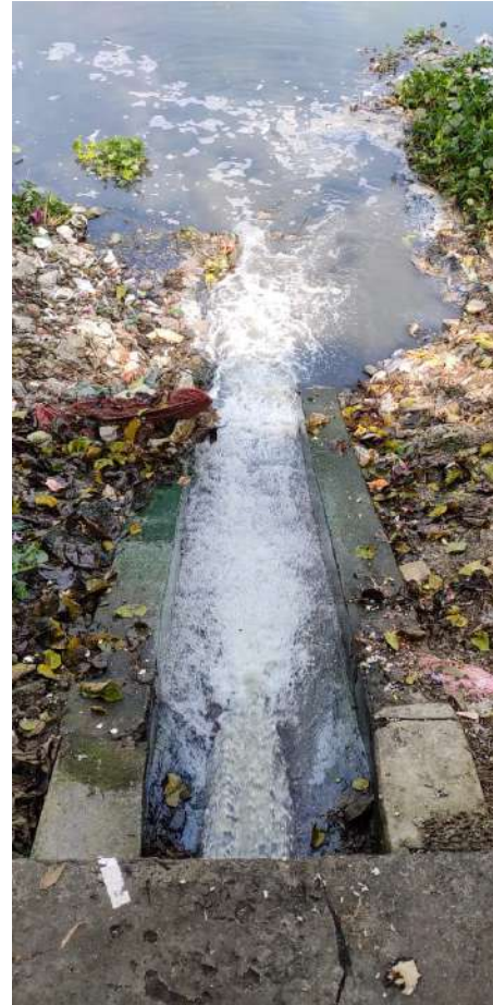
Outfall falling into Jalangi River
