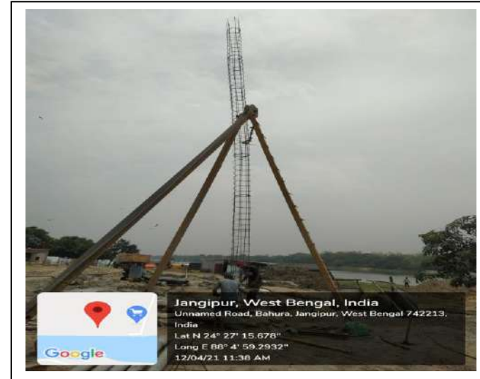
PILING WORK AT JANGIPUR STP SITE
