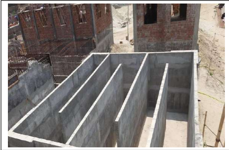
NABADWIP CHLORINATION CONTACT TANK
