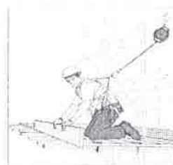
Worker harnessed to the scaffold component
