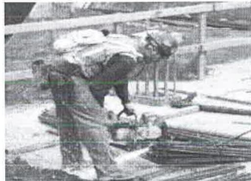
Cutting steel bars using electric saw
