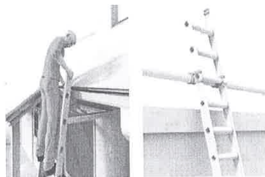
Securing ladder at top stiles and part way down
