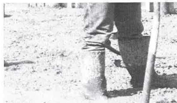
Wear gumboots while concreting
