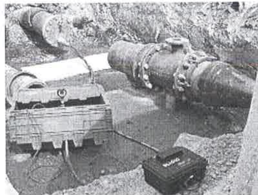
Pneumatic testing
