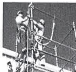
Worker harnessed to the scaffold component
