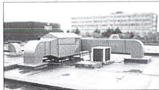
Mechanical means of ventilation
