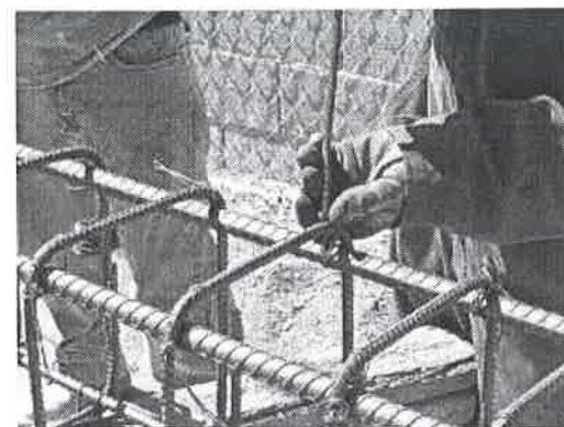
Heavy duty leather gloves to be worn while handling steel bars
