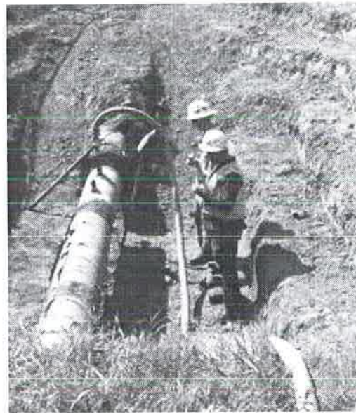
Hydrostatic testing
