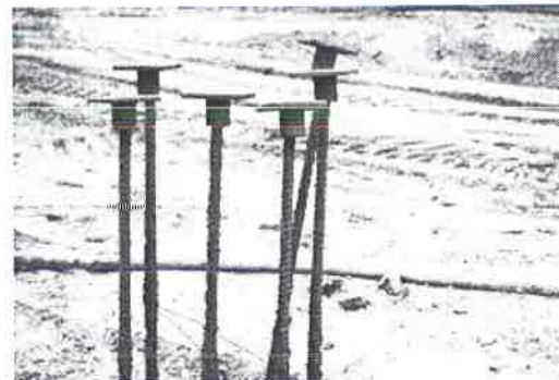
Reinforcement caps prevent cuts from sharp end of rebars
