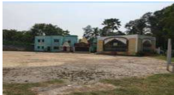
Temple & Recreational Centre near Arupara STP Boundary
