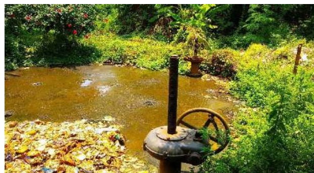
Grid Chamber at Arupara PS
