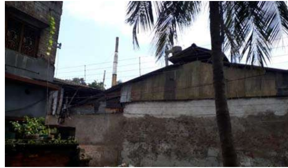
Industry behind the Aruapara STP with Stack
