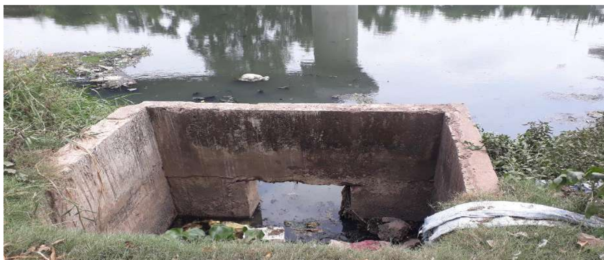
Figure 2.15 Outlet Point at Udaypur Canal
