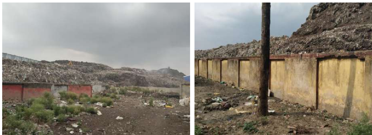
Figure 5.5 View of Baranagar Dumping Ground from STP complex
