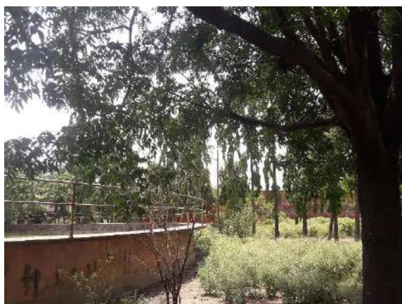
Vegetation near Clarifier Tank
