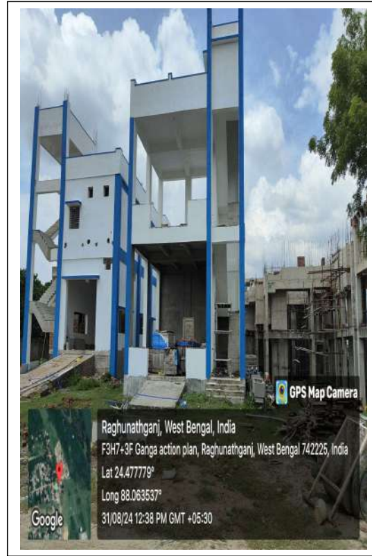
RAGHUNATHGUNJ STP SITE
