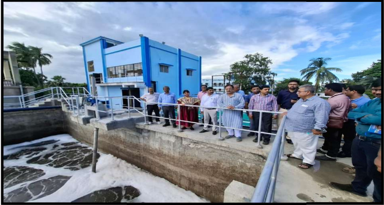
Photo of newly constructed STP at Sreenathpur, Ranaghat, Nadia
