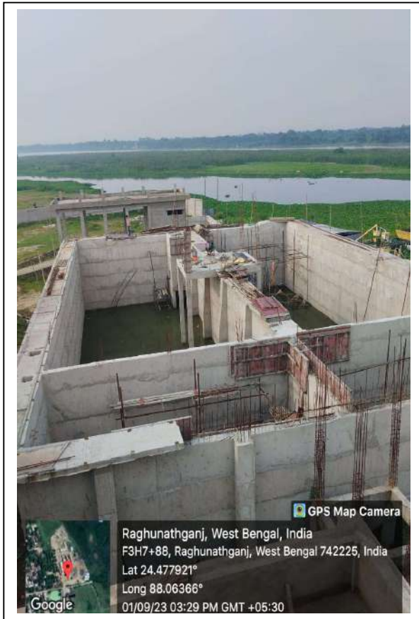
RAGHUNATHGUNJ STP SITE
