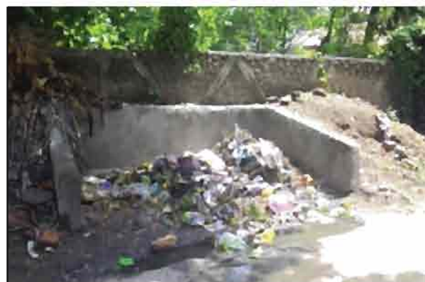
Masonry enclosure for dumping waste at local level at Tamralipta (Tamluk) Municipality
