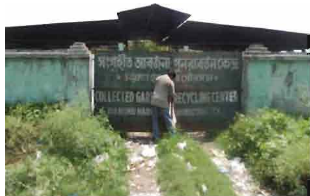
Material recovery facility at Diamond Harbour Municipality
